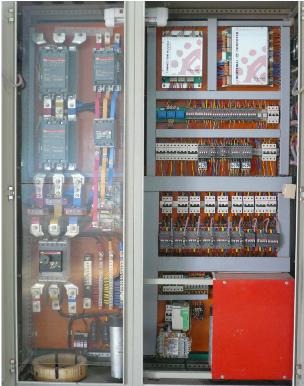
GENERAL ARRANGEMENT OF 250/80KW CONTROL PANEL
